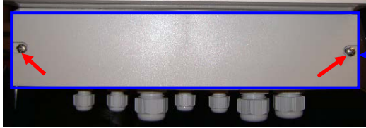
Picture 11 Removing cover plate from cable terminal
