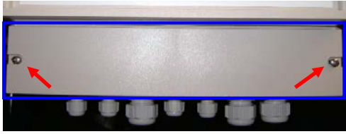
Picture 8 Removing cover plate from cable terminal
